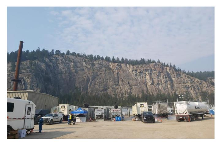
Temporary Generation Plant at Sheridan 2085S Shown here are the site office, 5 portable generators, a vaporizer, and one of the LNG Fuel trailers
