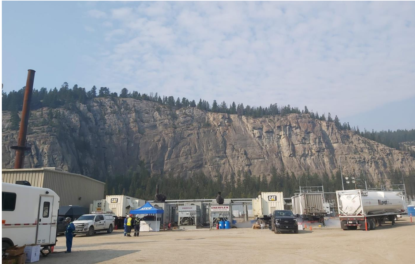
Temporary Generation Plant at Sheridan 2085S Shown here are the site office, 5 portable generators, a vaporizer, and one of the LNG Fuel trailers
